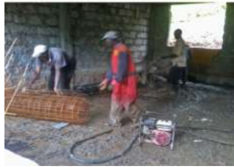
Reinforcing and pouring the concrete floor
